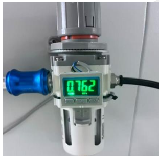
Main gas valve
